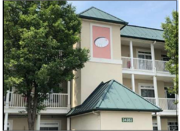
Example of metal roofing on multi-unit buildings
