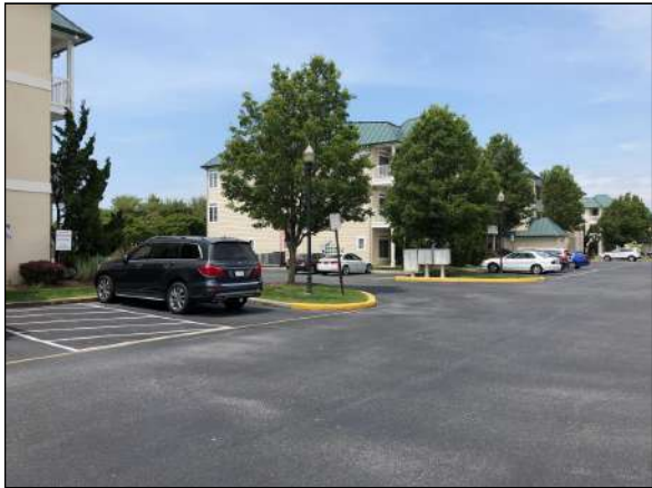
Asphalt parking lot
